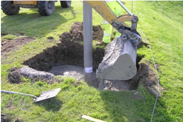
Direct burial installation as for steel posts.
