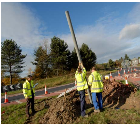
At 4.2kg per metre the 140mm post makes manual handling easy.
