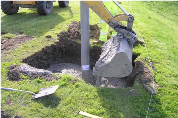
Direct burial installation as for steel posts.
